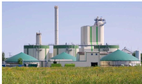
Anaerobic Digestion Plant
