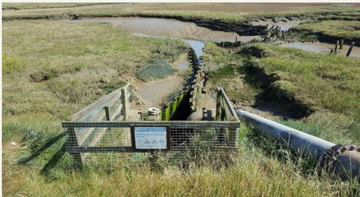
Kings Fleet sluice, the current discharge point to the salt marsh. The Felixstowe Peninsular project will now pipe water back to be used by farmers.
